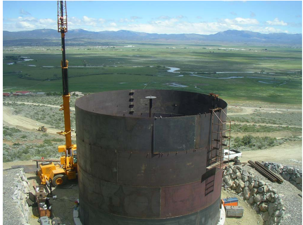
Eagle Ridge Water Storage Tank
